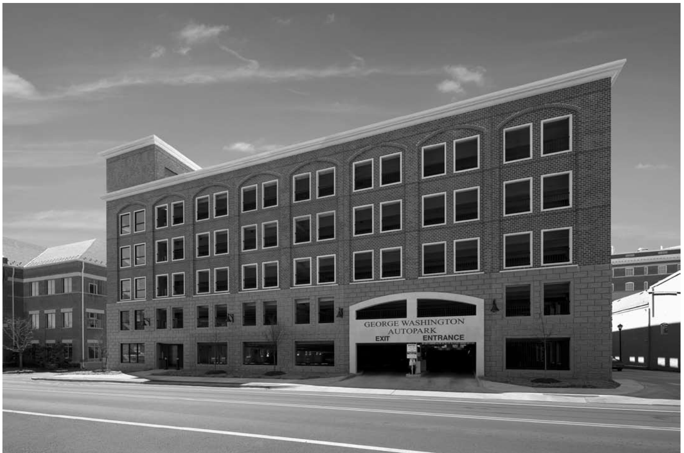
The 530-space, fully automated George Washington Autopark deck in Winchester was built using a public-private partnership. Photo by Eric Taylor Photography.
